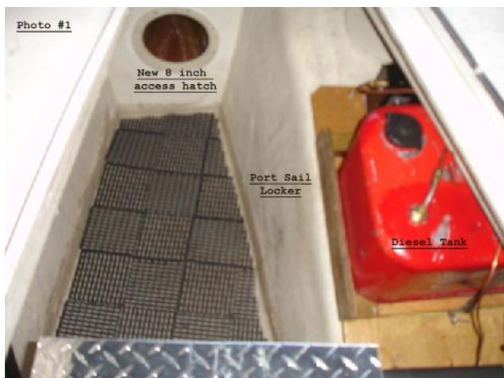
Photo 1. Installation of the fuel tank and the new eight inch access hatch in the port sail locker.
